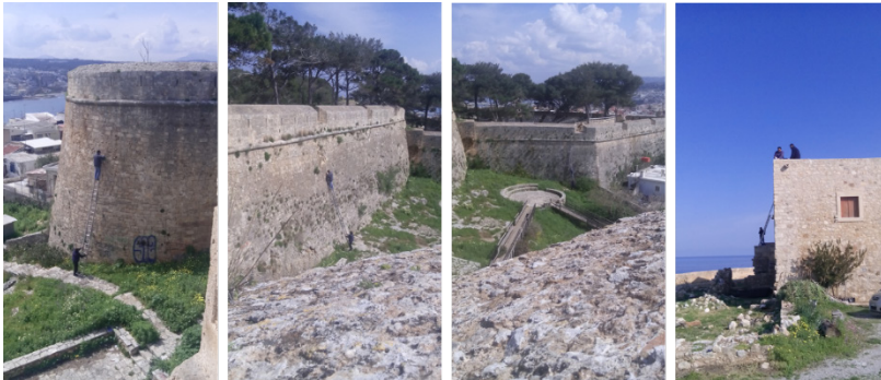
Figure 29. Images of the installation process of stable target references on the wall surface of Fortezza Fortress, Rethymno (Greece).
