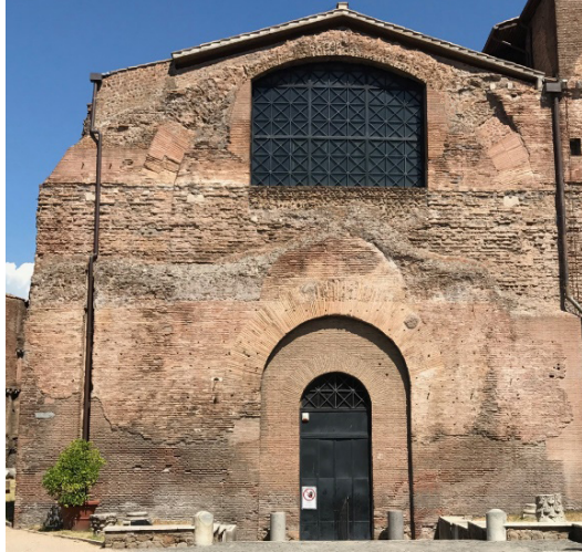
Figure 20. External wall of the Hall I, affected by rising humidity; the area chosen for monitoring is shown in red.
