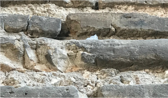
Figure 19. Wall of the Hall I, demonstrating the low aesthetic impact of FBG glued by silicone.
