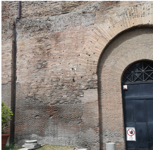
Figure 1. External wall of the Hall I, Baths of Diocletian Pilot Site, where is possible to see Rising Humidity, monitored by FBG sensors (almost invisible to a naked eye), connected to the computer inside the Hall, that can be remotely controlled.
